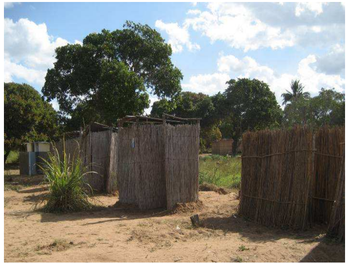
Pit latrines in schools in Gaza Province, Mozambique. (Photograph by Seung Lee)
